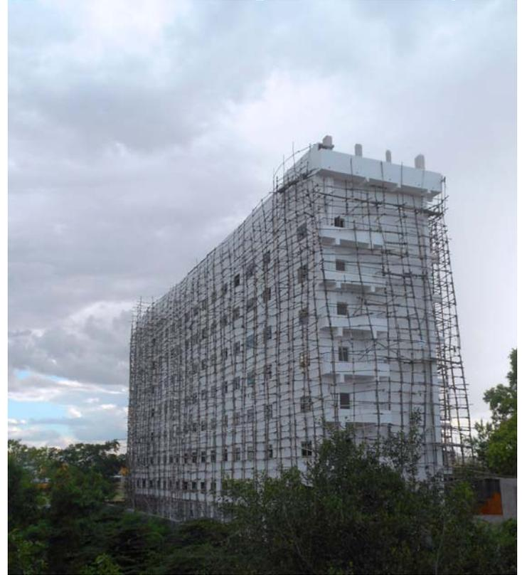
Nine stories of bamboo scaffolding, not tied in to the structure in any way I could discern!
