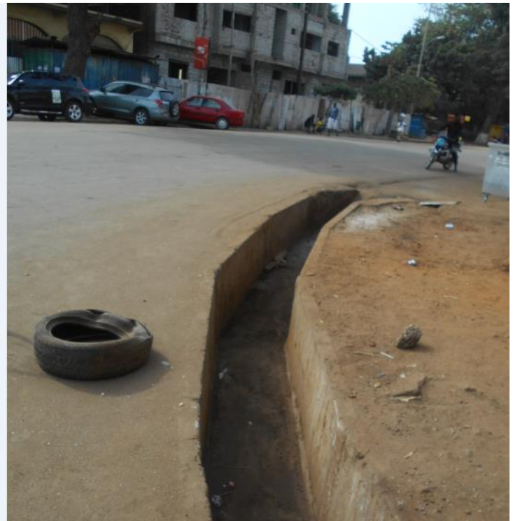
Empty gutters on street cleaning day. Road swept, all trash removed.
