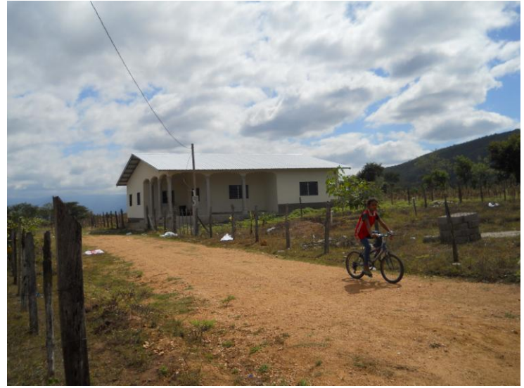
The Honduran Ministry of Health recently took possession of the new Punta Ocote clinic, an approximately 1800 square foot steel and concrete structure containing a pharmacy, general purpose room, and three examination rooms. It is staffed nearly daily by two Health Ministry nurses, and the majority of the funding (60%) was provided by the Salud Juntos partnership.
